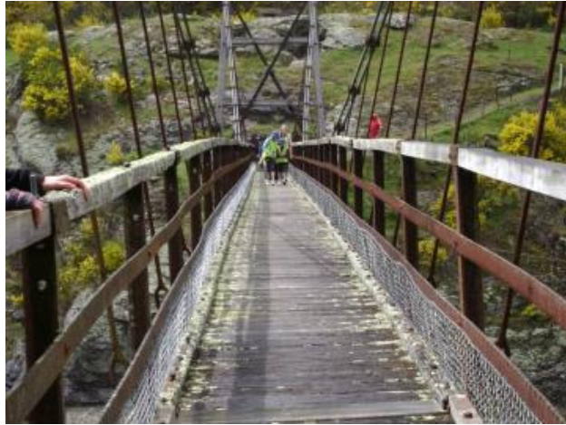
Horseshoe Bend Bridge
